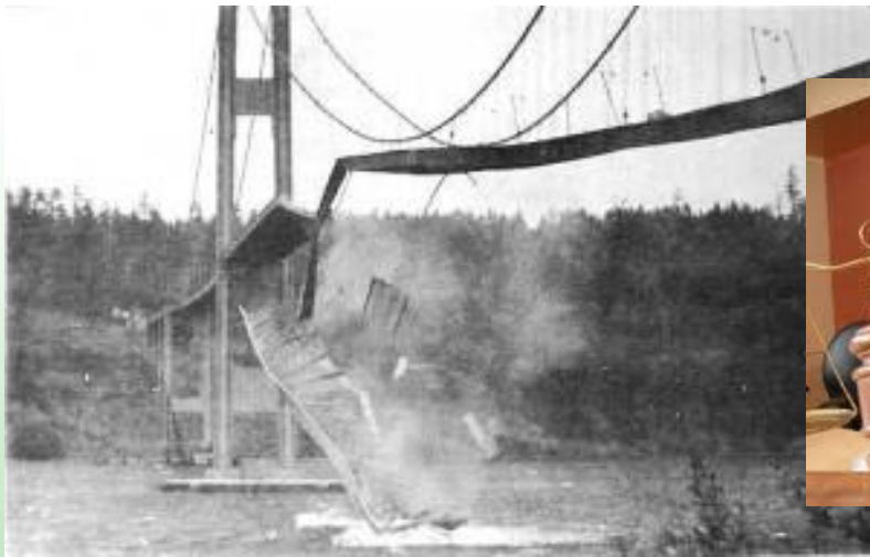
Galloping Gertie Bridge Collapse, by Allison Tatterson, Google images
